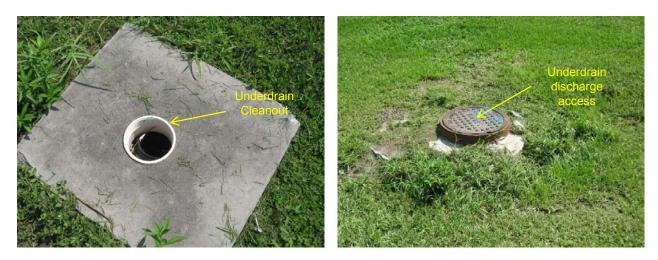
Underdrain Clean-out Structure
